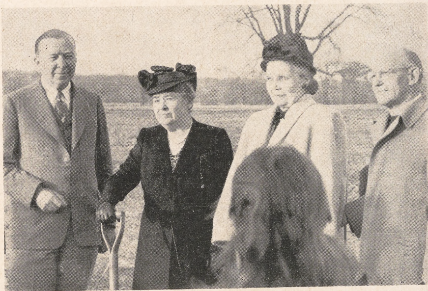
By the summer of 1949 Christ Church, Dearborn, Michigan, is to have a new $260,000 church. Ground was broken by Mrs. Henry Ford, pictured holding the shovel. At her right is Roy Bryant, her brother; Mrs. Stacey and the Rev. Hedley G. Stacey, the parish rector. Mrs. Ford donated the site for the new church.
