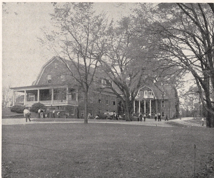
The Main School Building at St. Bernard's, Church School located at Gladstone, New Jersey.
